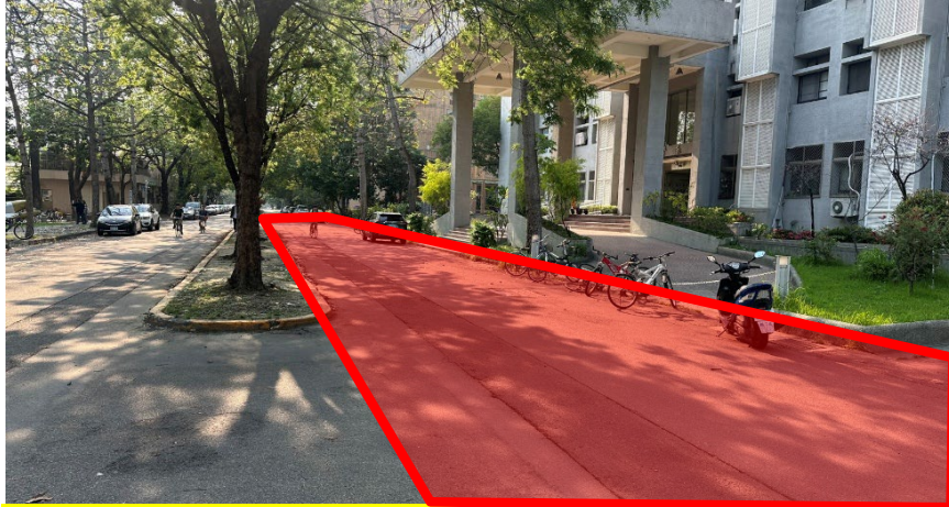
South side of the Chemistry Building
